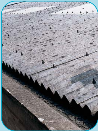
Asbestos cement roof
